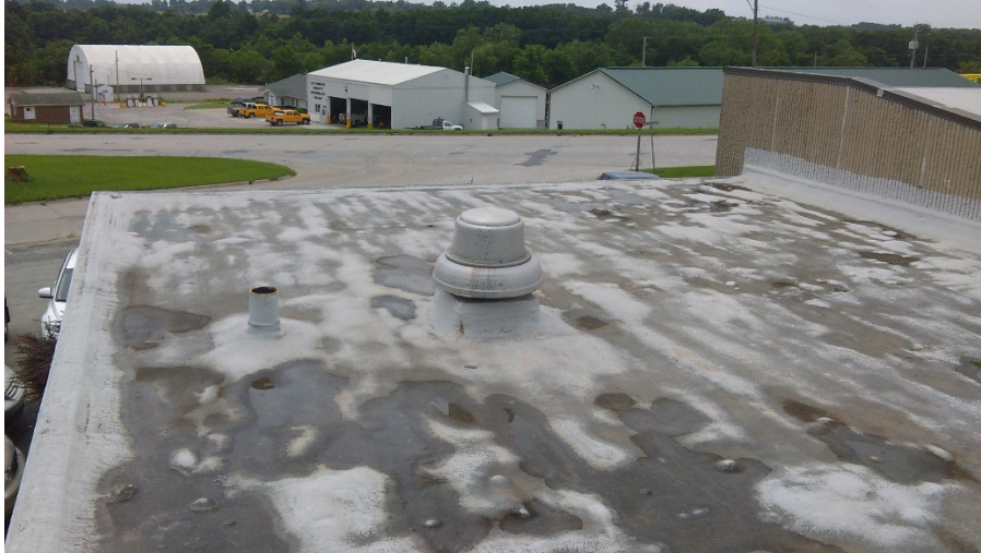
Figure 22 (Law Center Roof Failing, Spray-On Polyurethane system 'Bubbling' or Lifting from substrate)
